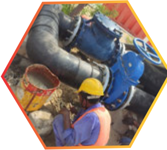
Installation of Hydrant at satwa Dubai project
