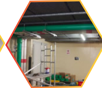
160 mm PPR pipes installation Ibis hotel al Rigga Dubai
