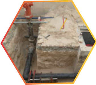
HDPE pipe installation for hydrant at Al qouz Dubai
