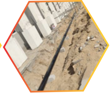
Installation HDPE drainage pipe line for sharjah government projects
