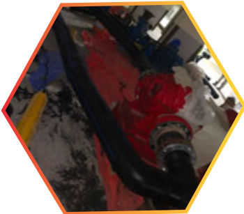
Installation of 200 mm HDPE pipes for flashing line
