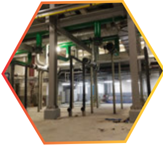
200 mm HDPE pipe installation work at Umm Ramool
