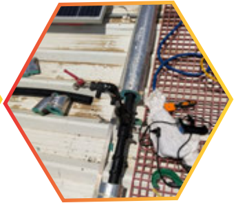
HDPE pipe installation work at Aramex free zone Dubai
