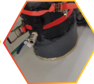
Hot taping connection branch saddle at Abu Dhabi post office tower.
