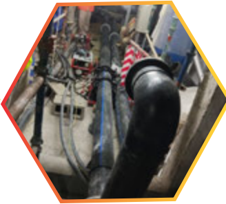
HDPE pipe installation work at Al Reem Abu Dhabi
