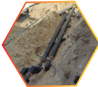
Chilled water pipe line installation at Sharjah villa project
