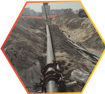
Installation of HDPE pipes at Dubai marine city
